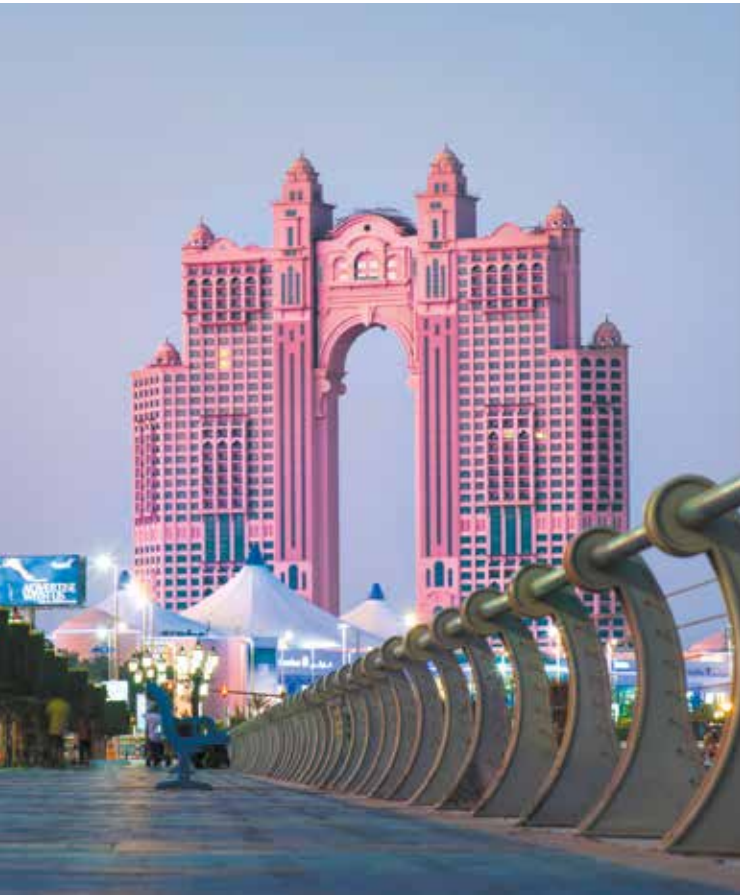
FAIRMONT HOTEL DUBAI - UAE - 2012 Heating/cooling system
