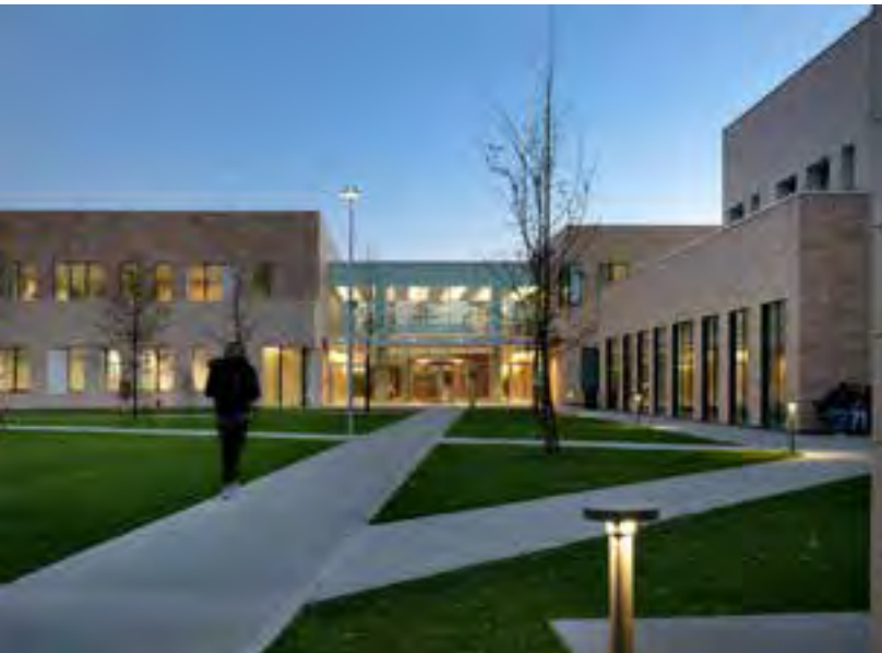
CAMPUS HUMANITAS - ROZZANO ITALY 2021 - Heating/cooling system
