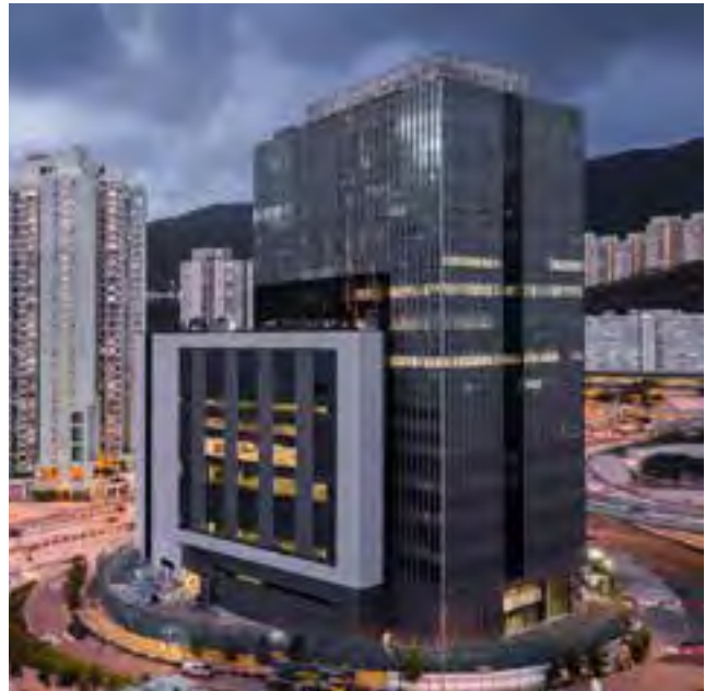
KOWLOON EAST REGIONAL POLICE HQ1 - HONG KONG CHINA - 2022 - Heating/cooling system
