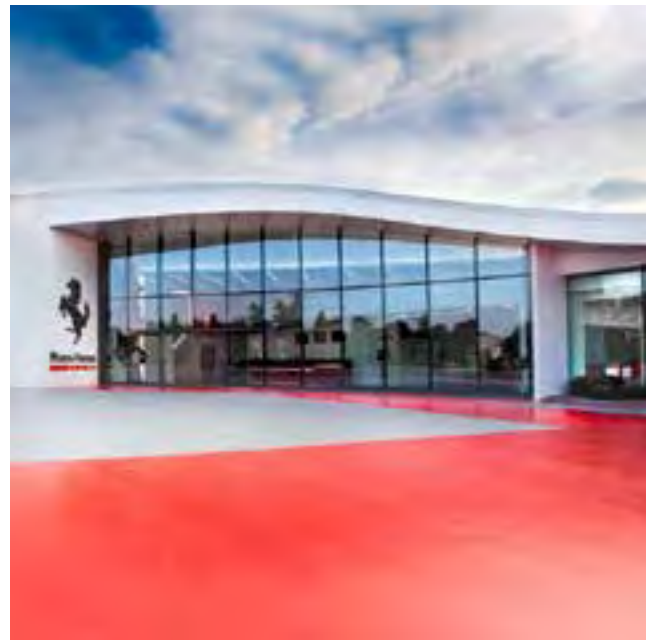
FERRARI - MARANELLO ITALY - 2020 - Heating/cooling system
