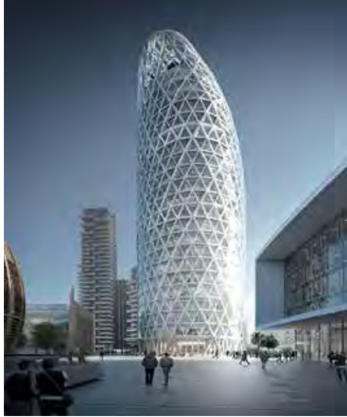
TORRE UNIPOLSAI - MILANO ITALY - 2023 - Central heating/cooling
