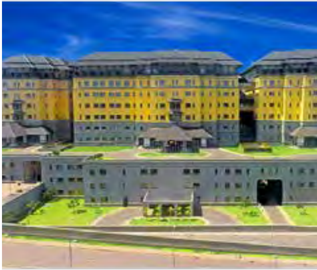
DIFENCE HEADQUARTERS – AKUREGODA COLOMBO – 2021 Heating/cooling system
