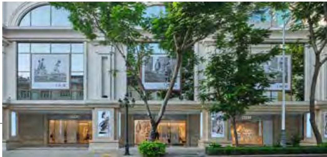
DIOR BOUTIQUE - HO CHI MINH CITY VIETNAM – 2021 Heating/cooling system
