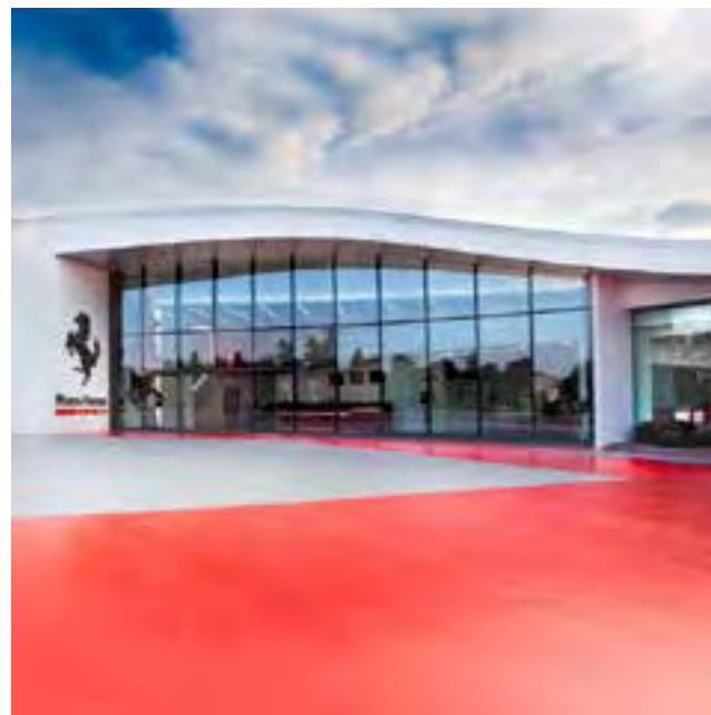
FERRARI - MARANELLO ITALY - 2020 - Heating/cooling system
