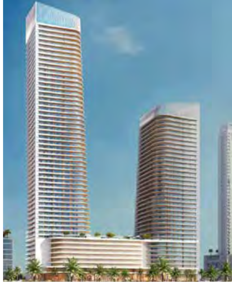
GRAND BLEU TOWER – DUBAI UAE – 2022 - Heating/cooling system
