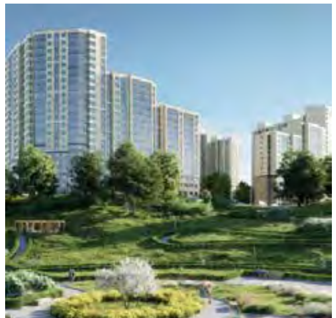
NEW KOTELNIKI RESIDENCES - MOSCOW RUSSIA - 2022 - Heating system
