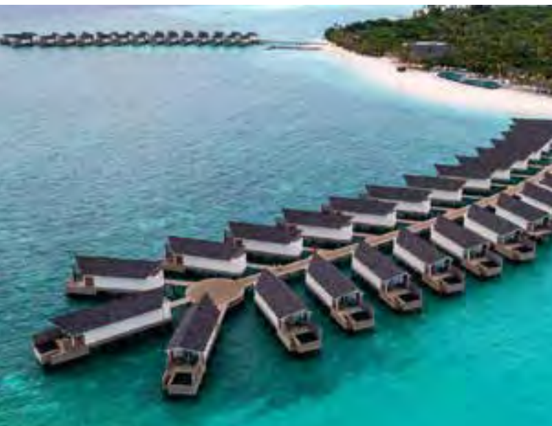
OZO RESORT - KUDAKURUTHU MALDIVES - 2021 - Water supply system
