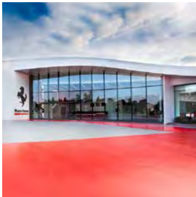
FERRARI - MARANELLO ITALY - 2020 - Heating/cooling system
