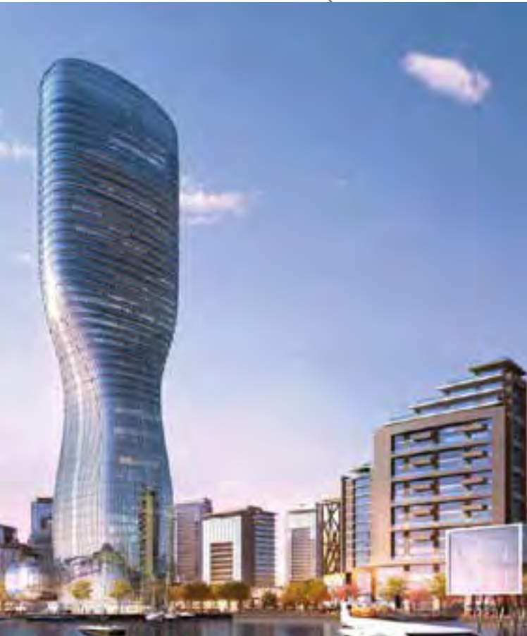
KULA TOWER - BELGRADE SERBIA - 2022 - Heating/cooling system
